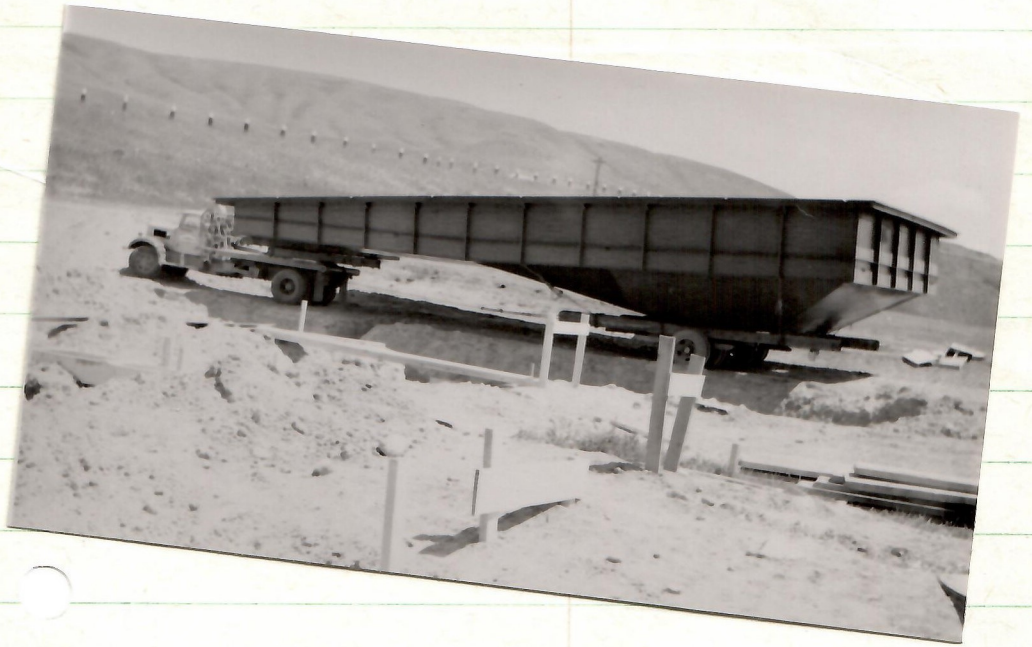
Swimming Pool 1960 under construction
